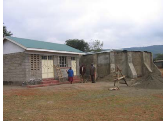
The Maai Mahiu borehole, pump house and water reservoir nearing completion.
